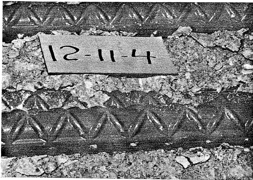
Figure 3.4 Coated Bars After Test
